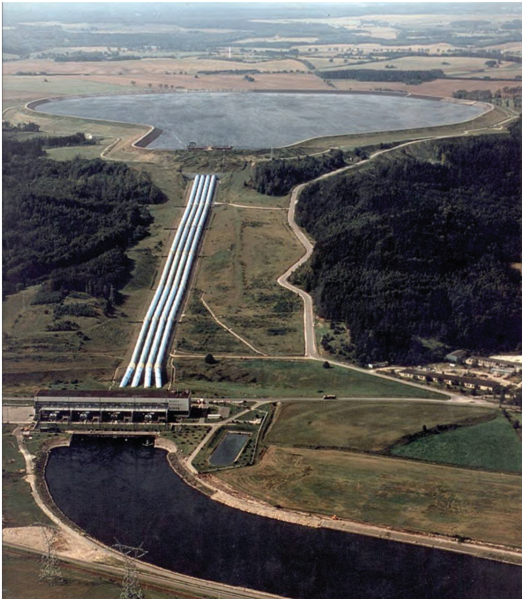
Fig. 1. Aerial view of Żarnowiec hydropower plant (Brochure, 1998)
